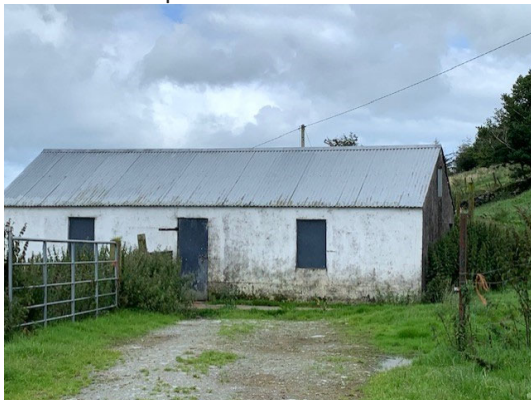
5. Single storey outbuilding
