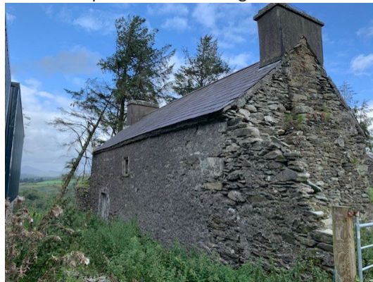
4. Rear and side view of disused dwelling showing exposed stonework
