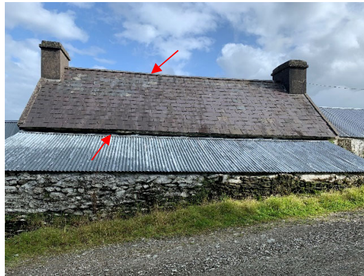
2. Rear view of dwelling indicating potential access points in raised ridge tiles and soffit
